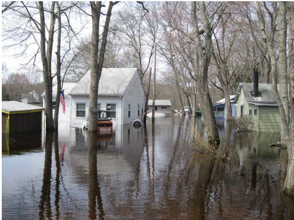
Figure 12: Inundation from flooding along the Pawcatuck River along Route 3 in Hopkinton, RI. (WFO Taunton Storm Survey photo)
