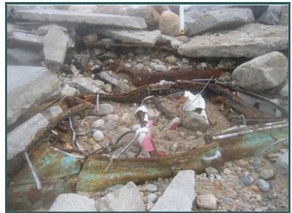
Above: A car frame, used to strengthen the dune system in 1957, was uncovered during Sandy.
