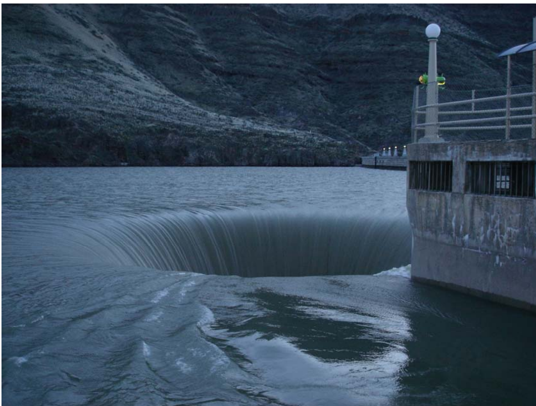
Figure 2. Water flows through glory hole spillway at Owyhee Reservoir in April 2006.
