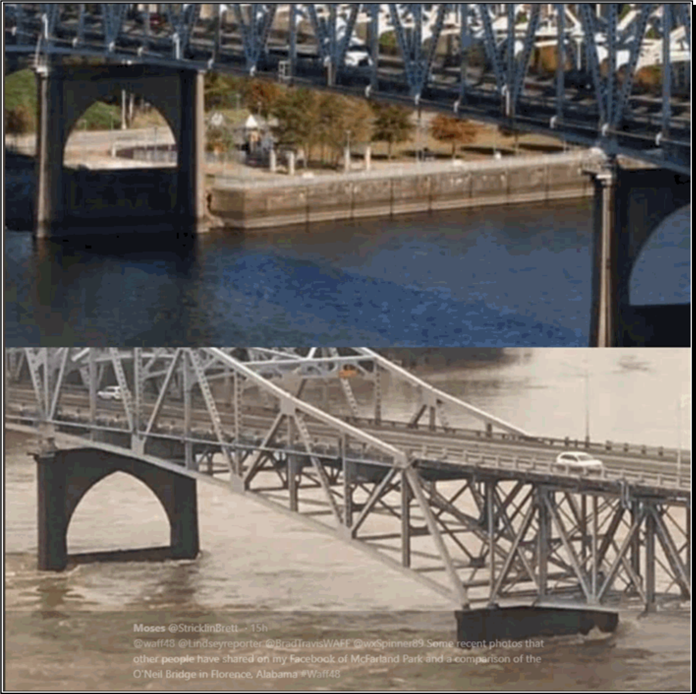
Photo shows McFarland Park beside the TN River at Florence river gage. Comparison is during the flood event at crest 2/24/19 and under normal conditions. Portions of the playground in the photo had nearly 10 feet of water over them.
