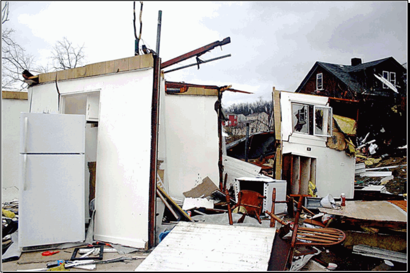
One of the homes that was significantly damaged in Uniontown, Fayette County Pennsylvania on Feb 15th. From the Herald-Standard.
