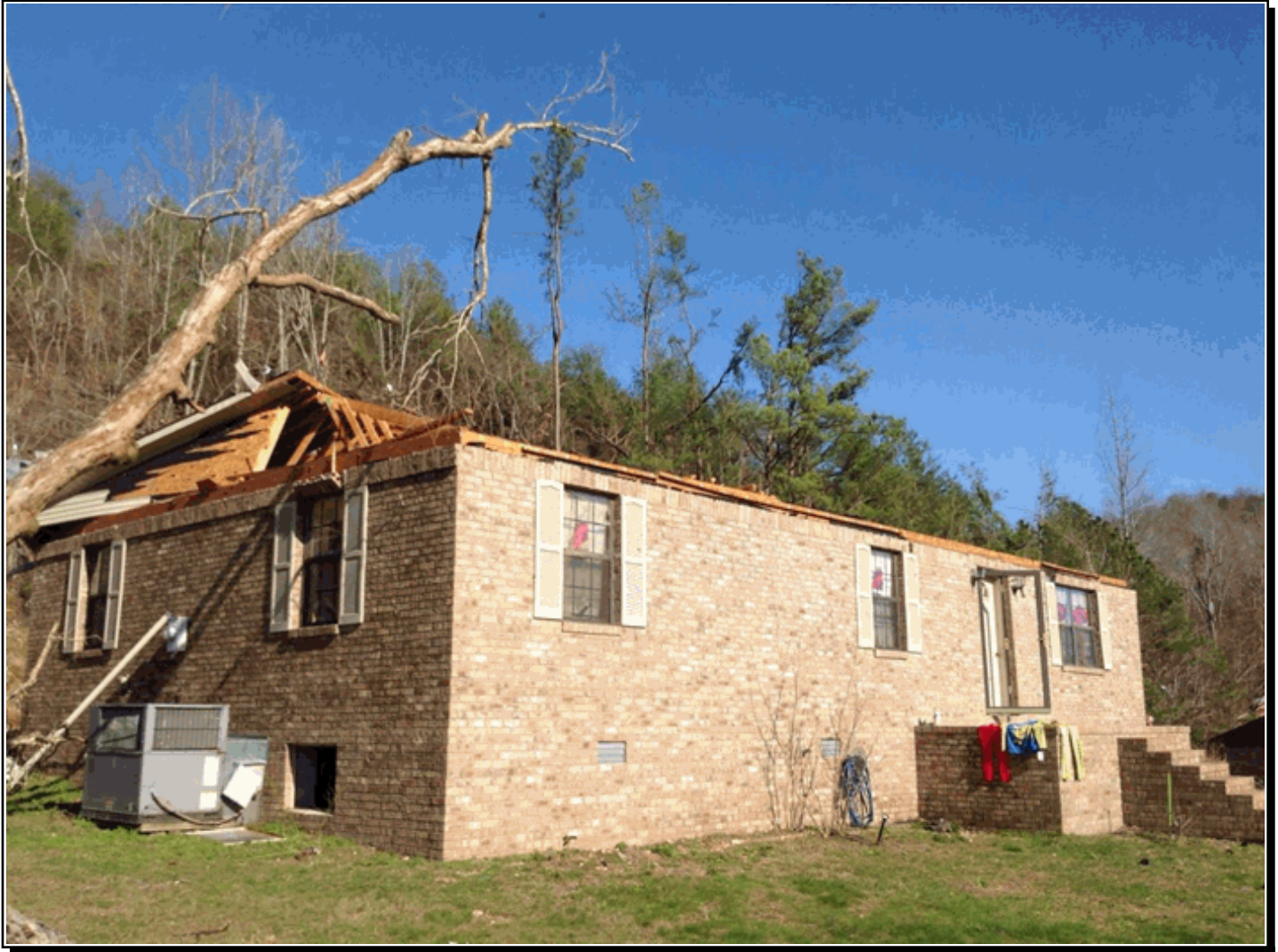
EF-2 damage. Roof of small house was removed/destroyed with walls still standing. Estimated winds ~115 mph
