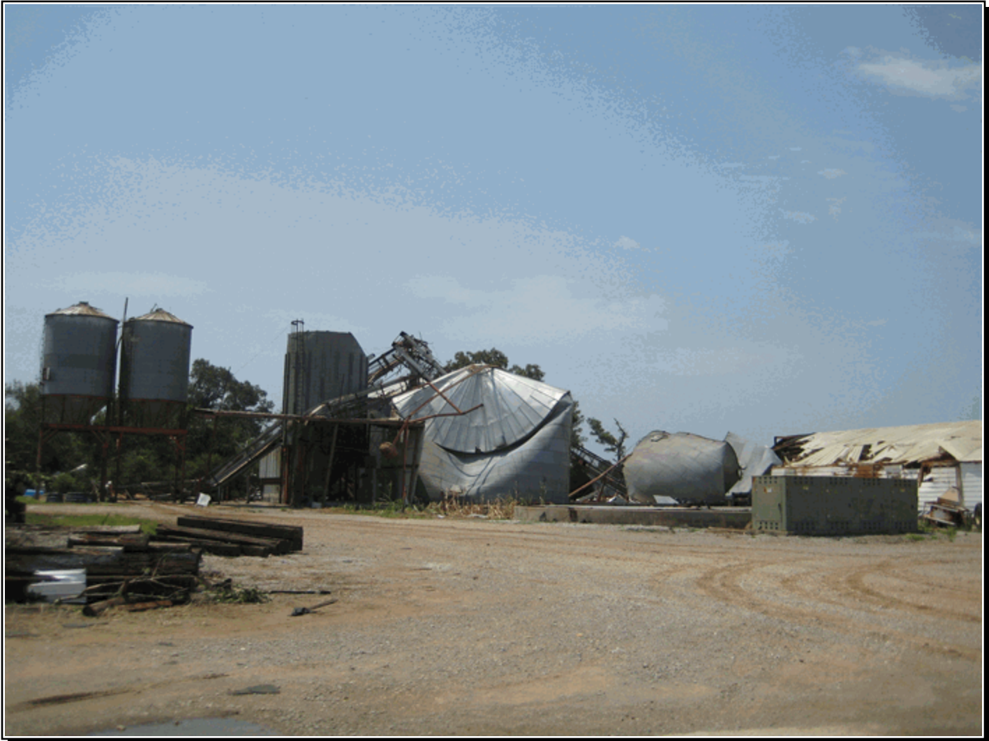
Grain silos crushed by microburst winds outside of Moulton.
