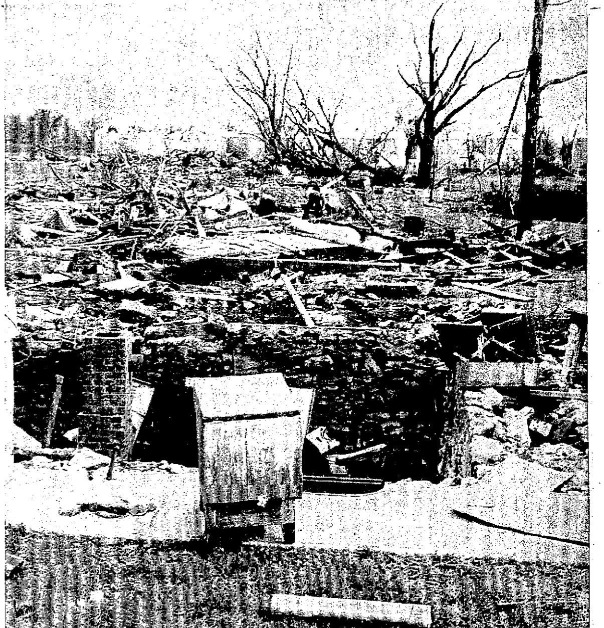
TWO DIED HERE —Maynard: The above basement walls are the only remains of three homes south of Iowa 150 near the Maynard Co-op where three-year old Glenda Kelly and Mrs. Louis Ponsar died as a result of injuries received from flying debris smashed about by the twin twisters. Glenda's mother, Mrs. Gordon Kelly, and her three small sons were severely injured in the tornado and rushed to hospitals in the area. Hundreds of others were injured in similar incidents throughout the area.
