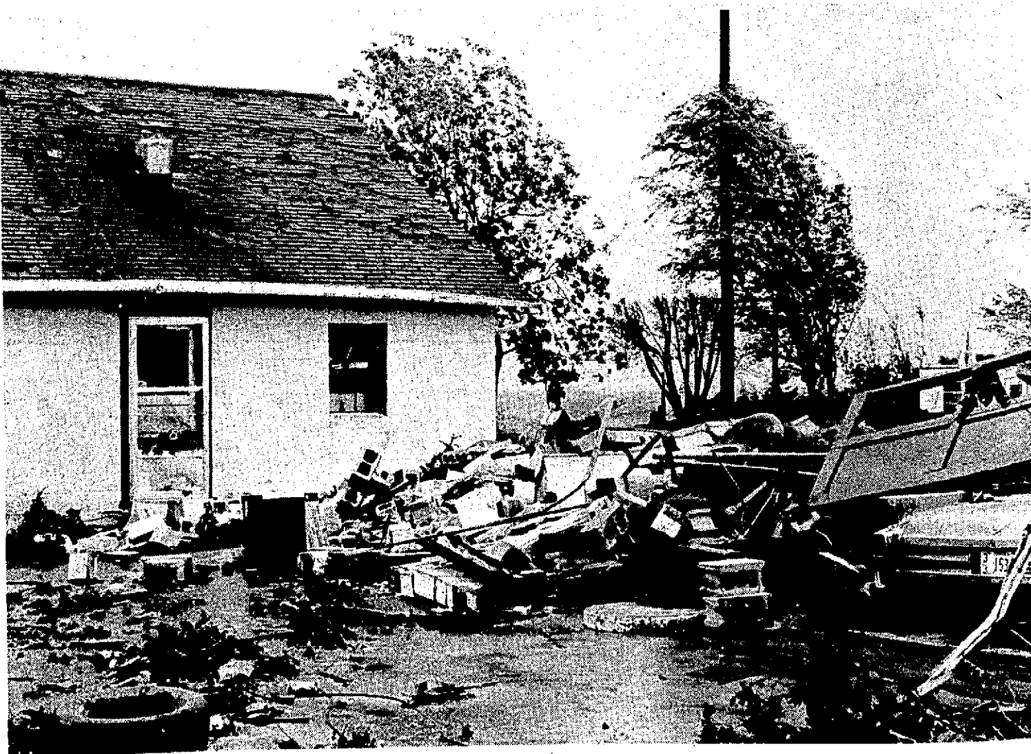
THIS PILE OF DEBRIS was piled between Baker's Blue Haven Cafe and Barney's Texaco at the north edge of Oelwein. Numerous sections of the city were blocked with fallen trees, downed power lines, roofing material and other barriers.
