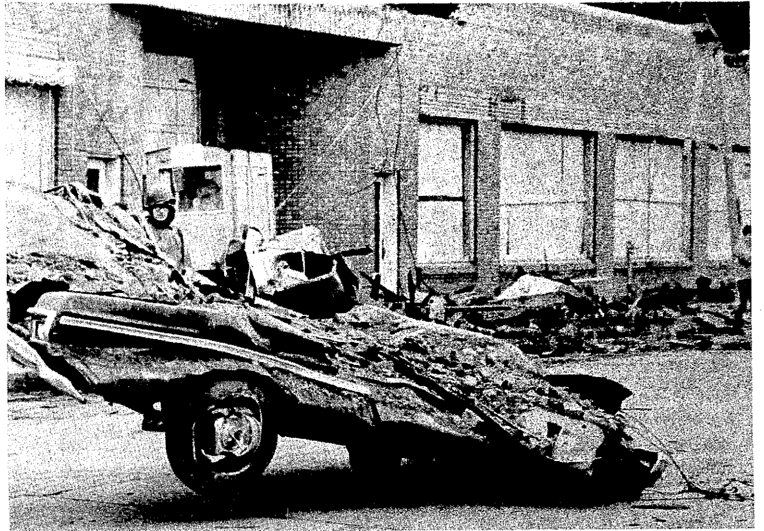
A GRIM EXAMPLE of the power in Wednesday's storm is this picture of a vehicle being towed away. The car was flattened by bricks and debris from a nearby building. Heavy automobile damage was reported throughout Oelwein along with an uncountable number of homes damaged in the storm.
