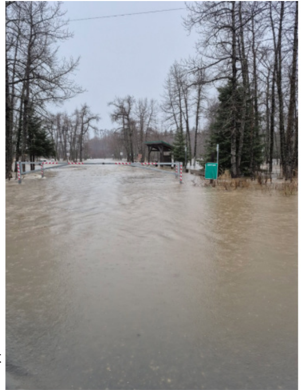
Flooding at the Anchor River Campground at the end of January 2025. Image courtesy of AKDOT
