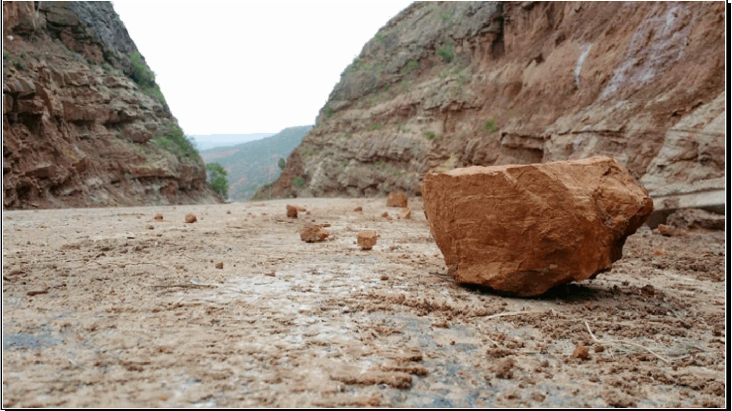
Mud and boulders were swept onto Highway 207 near the scenic overlook of Palo Duro Canyon by flood waters. Picture courtesy of KAMR Television in Amarillo.
