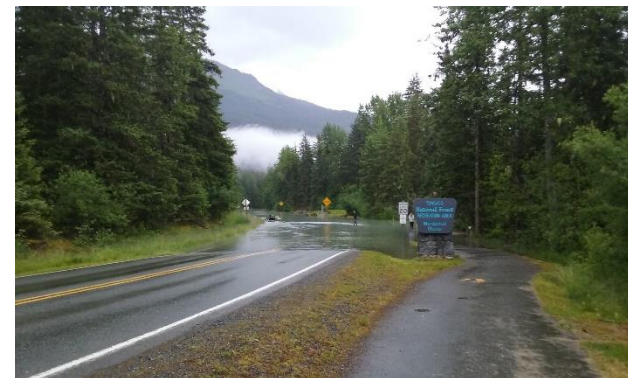
Flooded Roadway from a Glacial Dam Release
